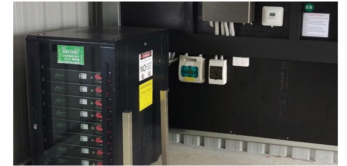
Rack-mounted lithium battery
