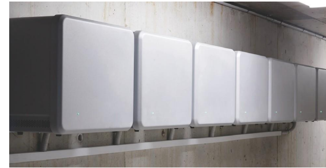
Wall-mounted lithium battery
